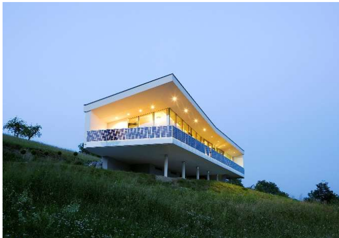
Kaltenegger Architects, Eisenberger
