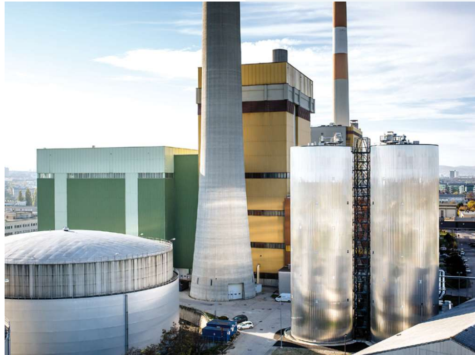
Photo: Wien Energie GmbH, Ian Ehm (from the Storage Initiative Report)
